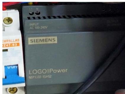
**Gambar 11.** PSU Siemens
